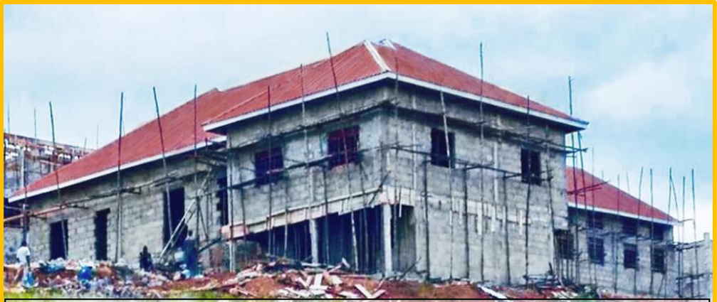
May 31: Dining hall roof is complete
