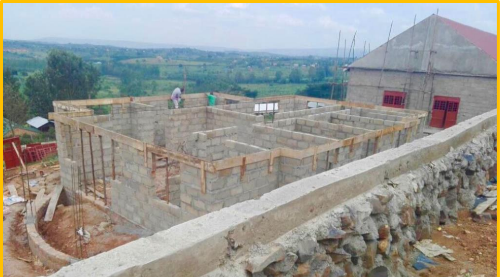
Admin. bldg going up next to dining hall
