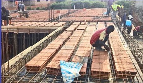
Closeup pictures of the maxpans onto which the cement (that will be both the top of the ground level & floor of the second level) is poured & smoothed. This is accomplished without any big cement mixers!!
