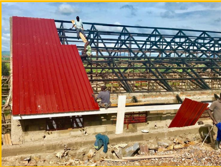
Below: Steel roofing is added to dining hall after the rafters have been sealed (May 22, 2018)
